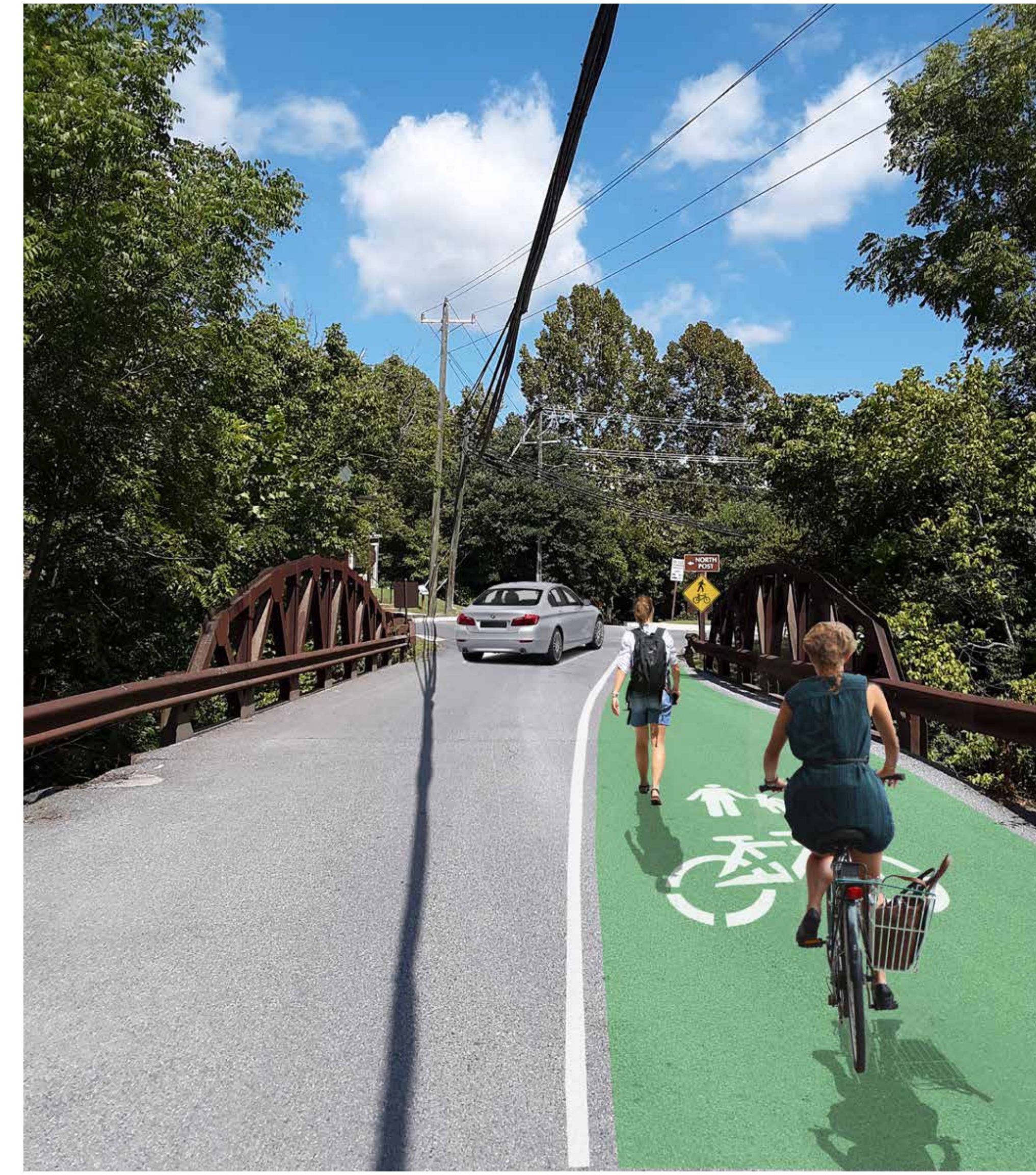
After: Bridge at Park Entrance with a one-way 14' driving lane and 8' bike/ped path
