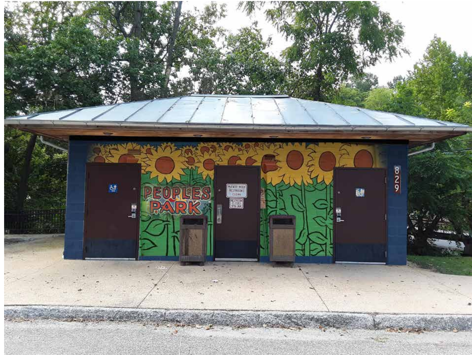
After: Mural on restroom facade
