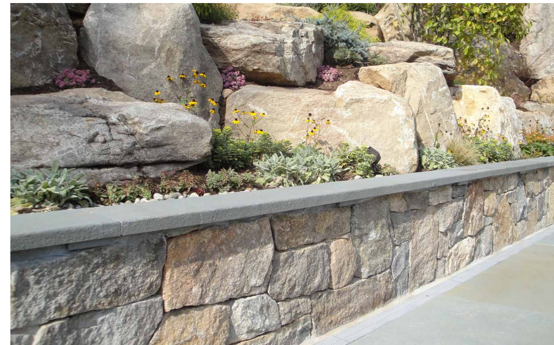
Seat wall at sign plaza
