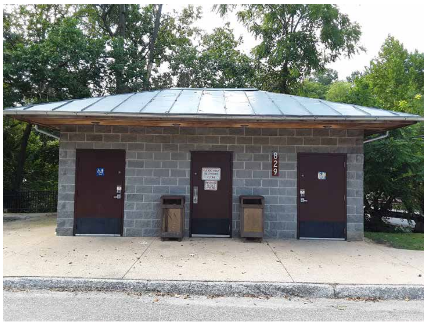
Before: Concrete block restroom
