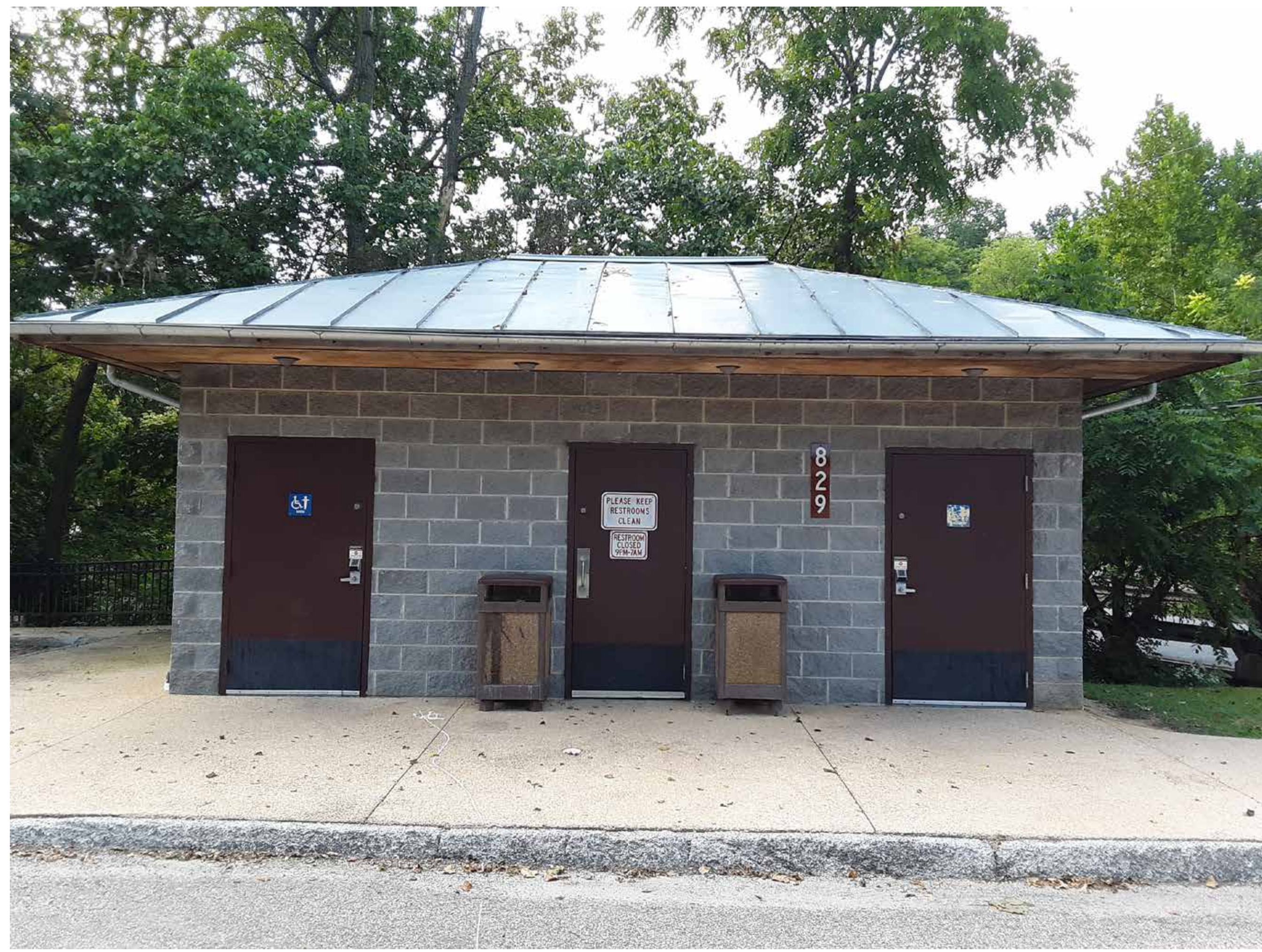
Before: Concrete block restroom
