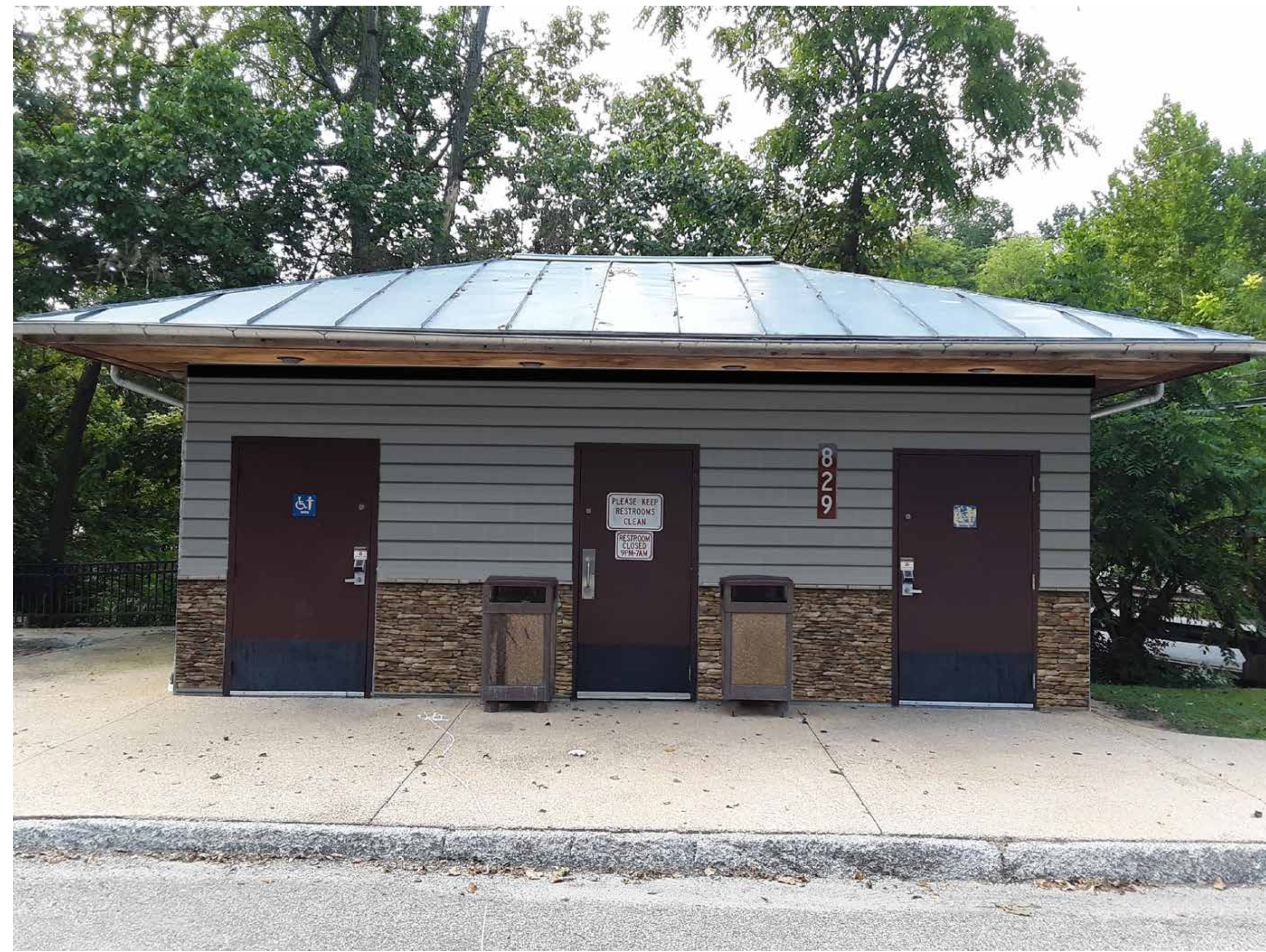
After: Cladding on restroom facade
