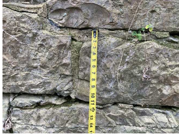
Figure 14 – Close-up view of the Dock Stone Masonry
