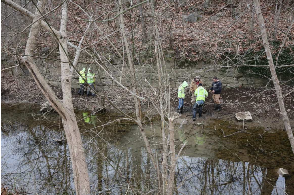
Photograph 3: Workmen digging two timbers.
