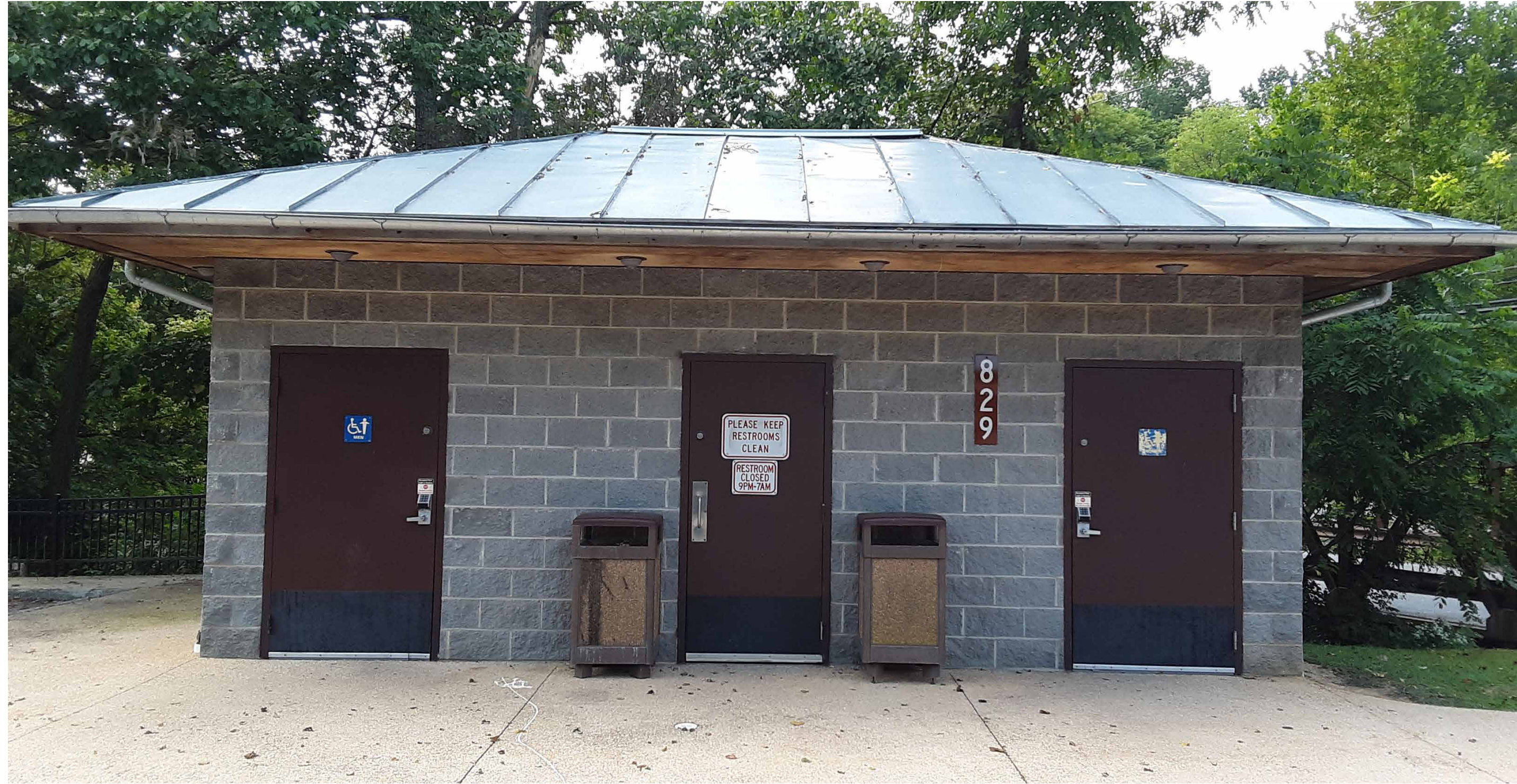
SS. Before: Concrete block restroom
