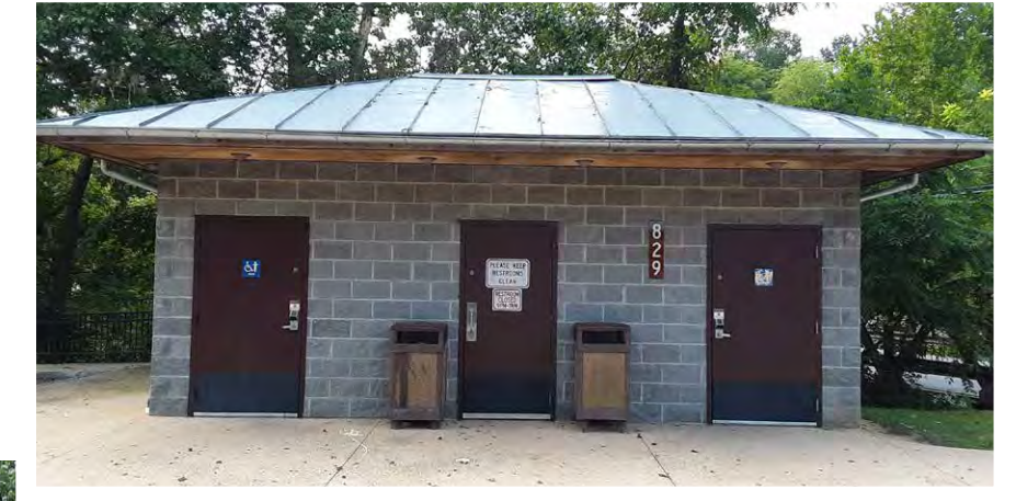
SS. Before: Concrete block restroom
