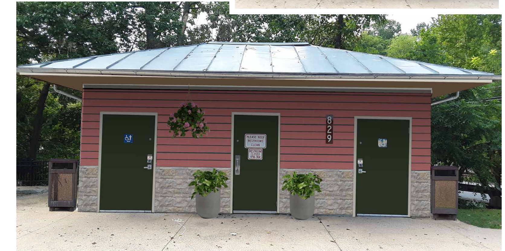
SS. After: Cladding on restroom facade, compatible with the Miller House
