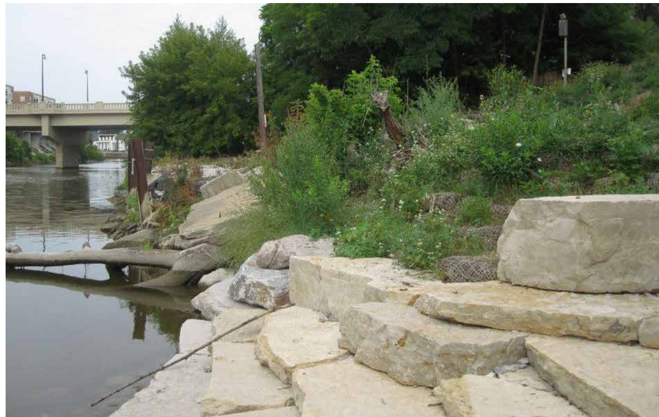
DD. Stabilized and re-vegetated river edge and fishing access
