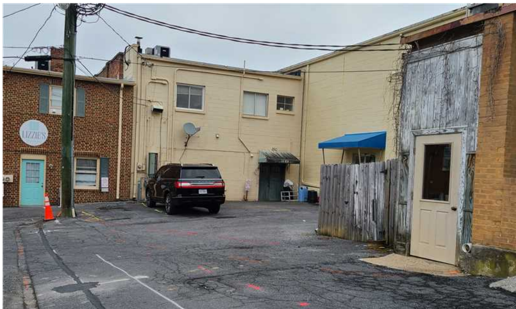
EXISTING REAR OF BUILDING
