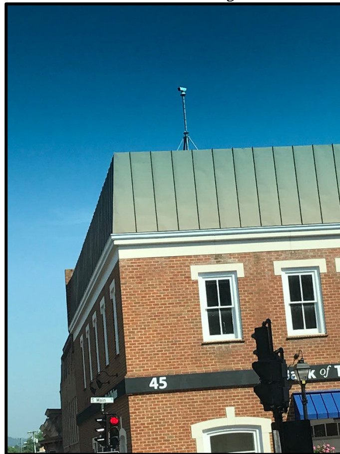
45 South Main Street existing conditions
