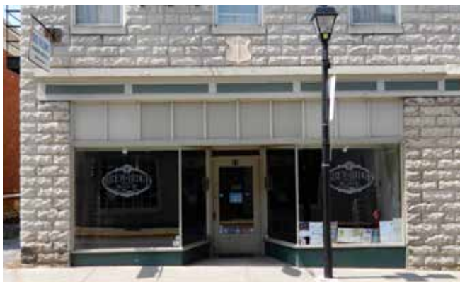
Early 20th c. storefront with essential elements. As often happens over time, the transom glass has been painted over.
