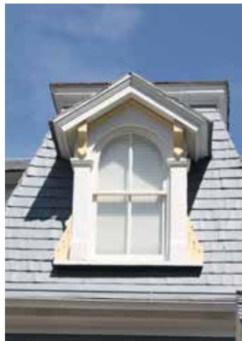
Four-over-four sash with arched upper sash in a dormer window
