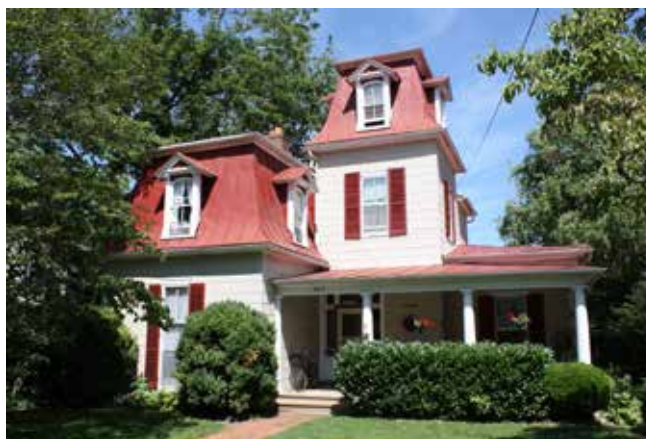
The trademark Mansard roof with its dormer windows on both the house and tower identify this style.
