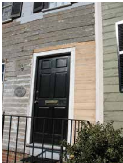
Only replace the sections of wood siding that are too deteriorated to repair.
