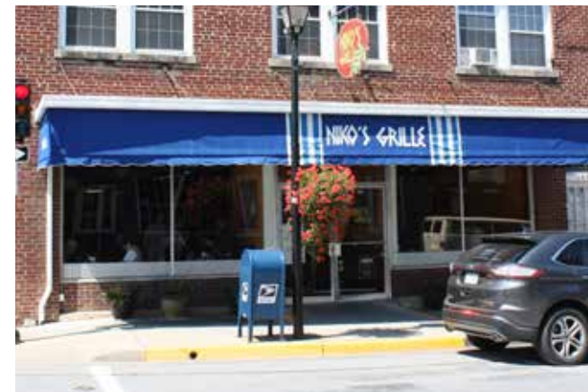
Flat canopies can also have fabric awnings that hang from the edge and provide space for signage.
