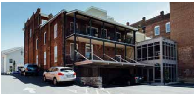
This rear addition in Lexington, VA consists of new balconies, green roofs, & a contemporary rear entry block.
