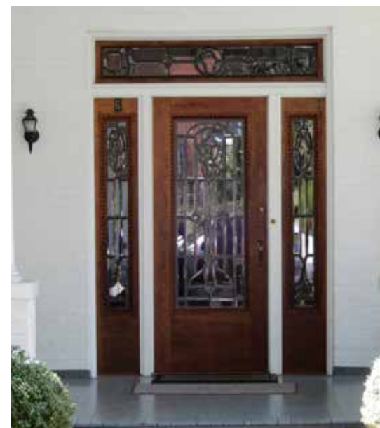
Leaded glass patterns on the door, transom and sidelights are an important decorative and character-defining feature to this entrance.
