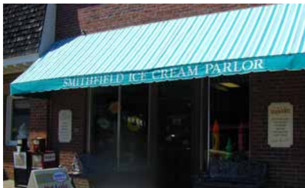
The valance of an awning can also be used for signage as shown in this example.
