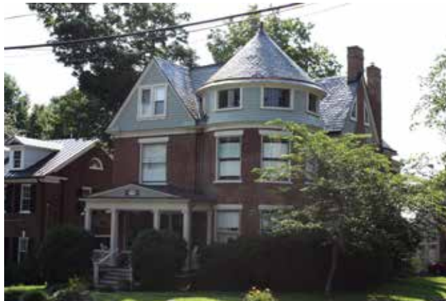
This brick Queen Anne has a prominent corner tower, tall chimneys, one-over-one windows with stone lintels and a partial front entry porch.
