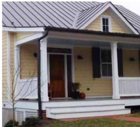
New materials like cementitious siding and a pre-coated metal roof create a traditional appearance on this new residence.
