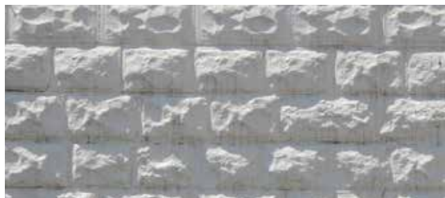
Early concrete block was molded to look like stone.
