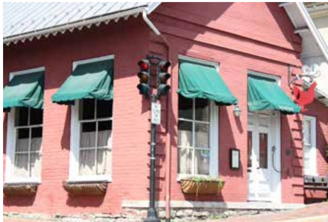
These retractable awnings on a north and east elevation can be pulled back to let in more ambient light when the sun moves to the west.
