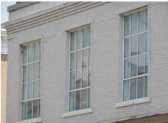
Steel windows are found on several commercial buildings in the district.
