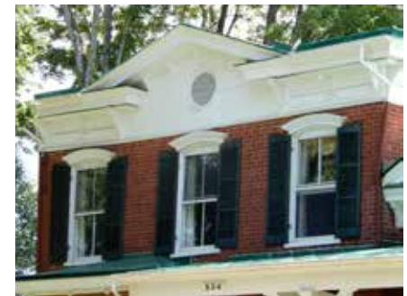
Decorative cornice brackets and window hoods are distinctive details on this Italianate house.
