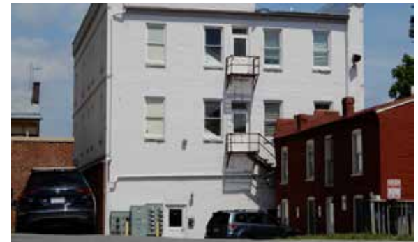
Utility boxes in this example are placed on the rear of the building, an appropriate location for such appurtenances.
