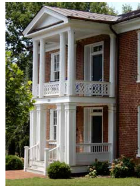
Brick houses typically have a single trim color with doors painted an accent color such as in this example.
