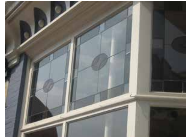
Stained glass designs were also used for transom areas of storefronts in the late 19th century. This is a contemporary interpretation of that application.
