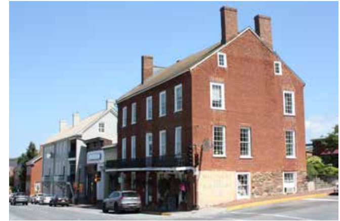
This Federal period brick residence has pairs of flanking interior end chimneys. Note the wrought iron balcony that was created when Main Street was lowered and the building's basement became the first floor with added storefronts.
