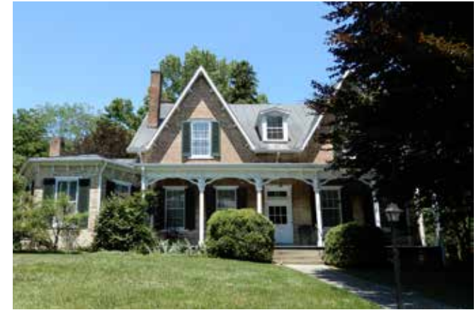
This brick residence shows the influence of the Gothic Revival with its matching steep gables and decorative bargeboards. The one-story decorative porch is typical of the period.
