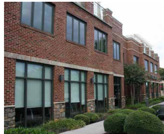
These contemporary windows in this new building use mullion dividers to reduce their larger scale.
