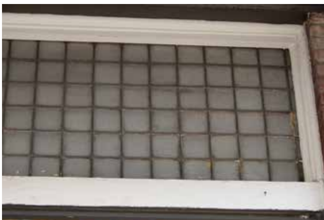
Prism glass panels are used in storefront transom areas to filter light entering the interior of the building's main level.
