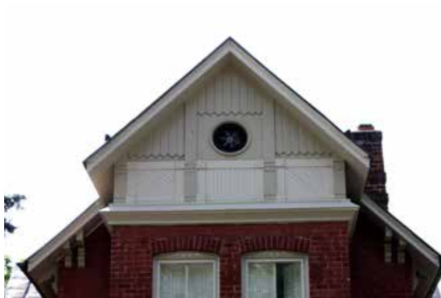
Wood is used to provide decorative panels in the gable end of this Victorian era house.
