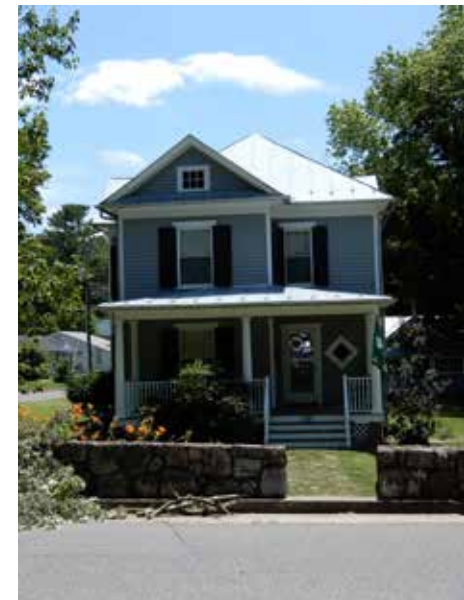
This simpler and smaller example of the Queen Anne is identified by its projecting gable intersecting with its hipped roof. Underneath its full width porch is a typical diamond shaped window next to the entrance.
