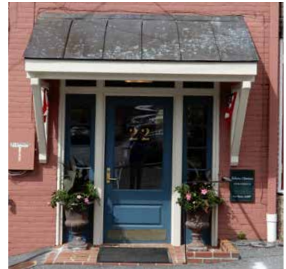
This rear entry is enhanced with a shed roof cover, and a new brick base at the door flanked by a pair of planters. A small wall sign identifies the business.
