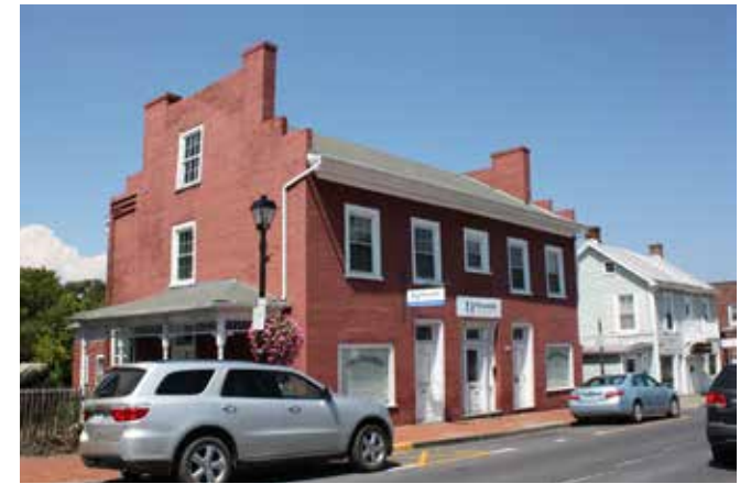
This early 19th century building has stepped gable ends containing two end chimneys. Later store windows likely were enlarged. Entrances contain transoms and the center one has sidelights as well.
