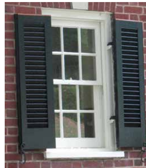
Any new windows with divided lights should have raised muntins; & shutters should be hung on pintels with hinges like this historic window example.
