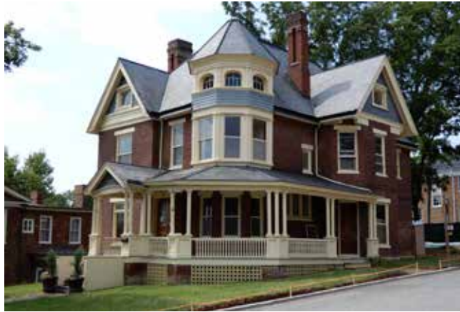
This large ornate example of the Queen Anne has a complex roof, corner tower, wrap-around porch and decorative chimneys, all attributes of this style.
