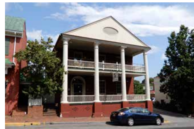
Brick is frequently used for foundations.
