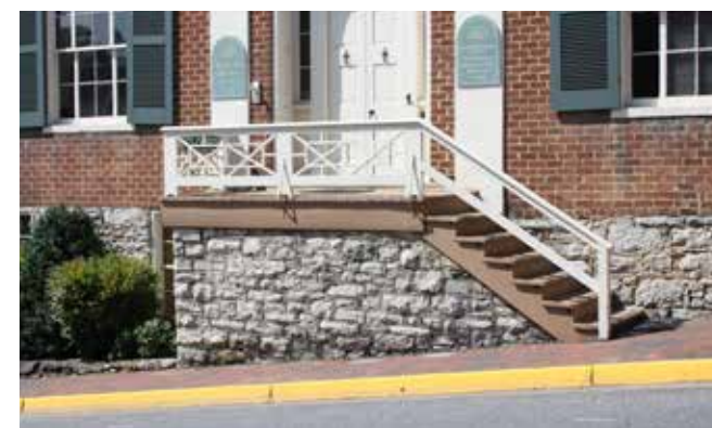
Stone, mostly local limestone, is also commonly used for foundations.
