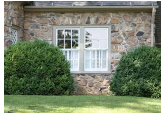
A double window made of a pair of six-over-six windows found on a 20th c. revival style residence.
