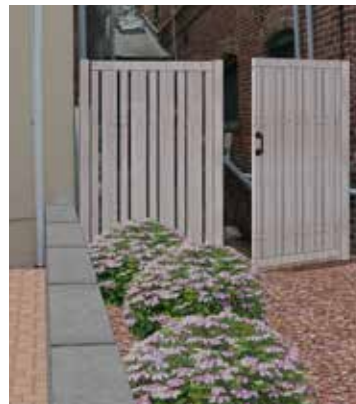
Other areas where site appurtenances are located should be screened with materials like this set of wooden gates if possible.
