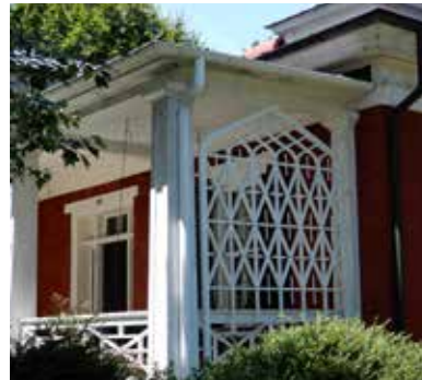
The decorative wood porch trim on this example is a series of Gothic & Tudor arched forms.
