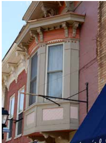
Frame bay windows can be found on both commercial and residential buildings
