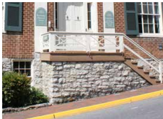
This house sits on a native limestone foundation. The surrounding site wall is also stone to match.
