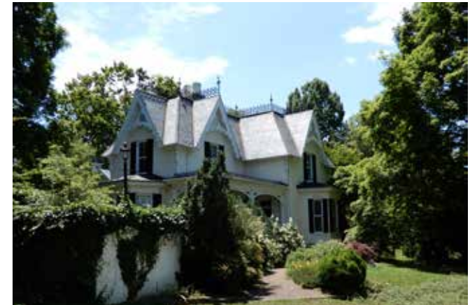
This larger domestic example shows the continuing influence of the Gothic Revival with its steep gables. Note the decorative slate shingle patterns, ornate roof cresting and bay window, also of the period.
