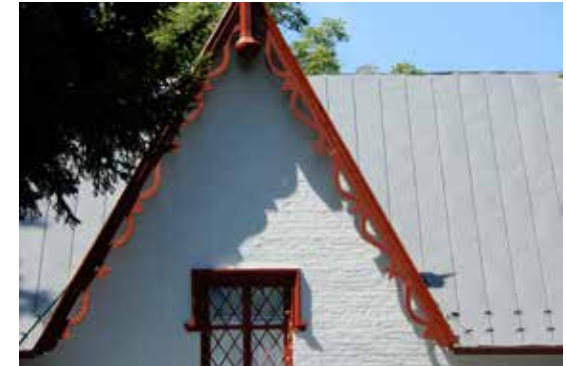
This steeply pitched gable is defined by the decorative rake board in the Gothic Revival style.
