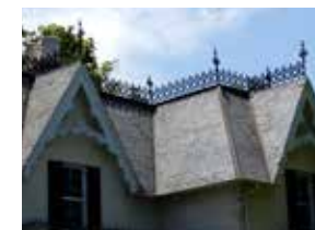
A decorative patterned slate roof has retained its metal cresting.
