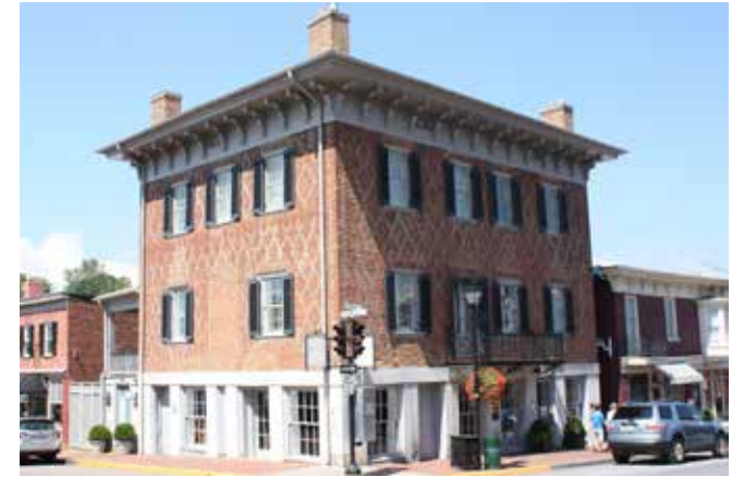
Lexington's most prominent Italianate cornice is on the Alexander-Withrow Building, an 18th century structure with a 19th century roof alteration. Note the original brick pattern of decorative diapering, a rarely used technique.
