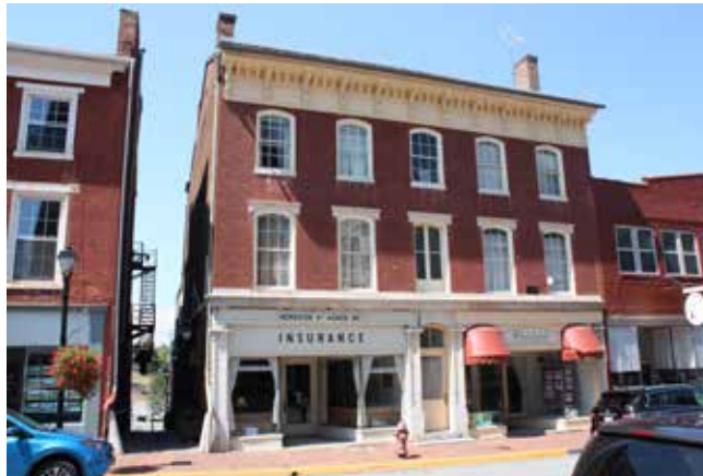
This well preserved example of the Italianate has the trademark bracketed cornice, segmental arched openings and its original central entrance to the upper level.
