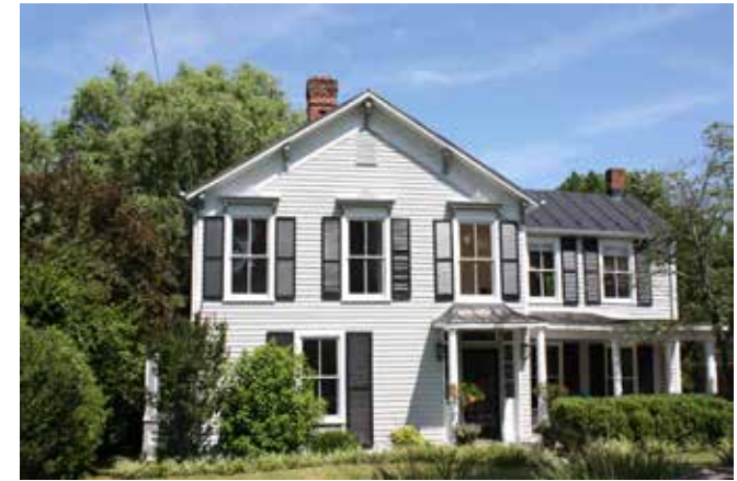
Wood window caps and a bracketed cornice are details on this “L” example.
