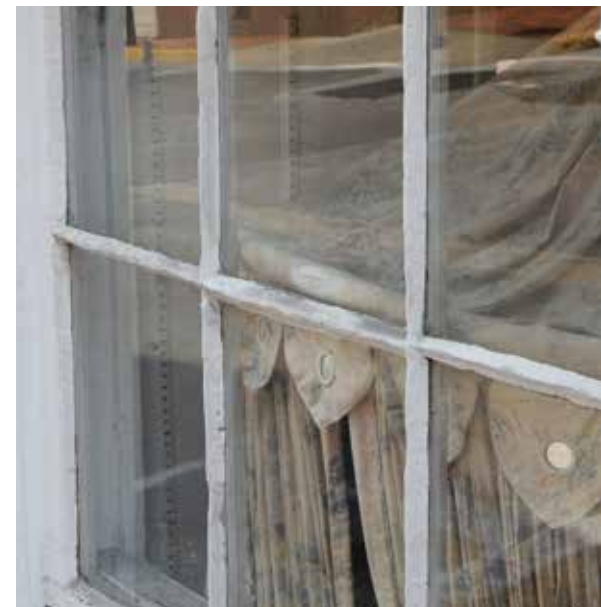
This original wood window retains its historic glass which adds texture and interest to the windows.
