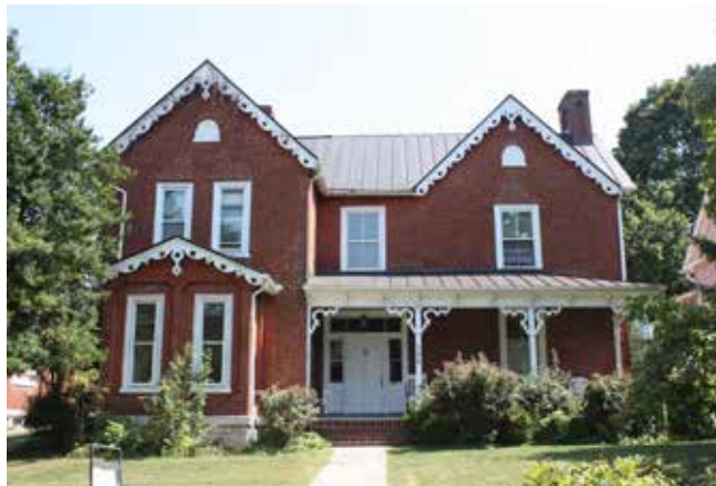
This brick example with its three decorative gables and porch reflects the continuing influence of the earlier Gothic Revival.
