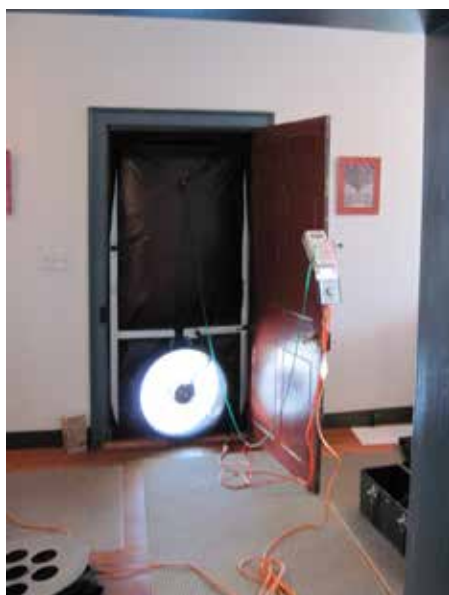
A blower door test is a critical step in an energy audit. It reduces air pressure in the building so that leaks can be found through temperature variations.
