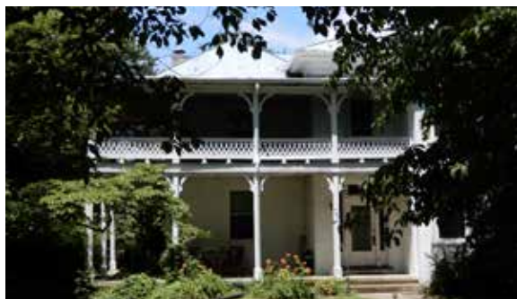
Two story porch with decorative wood balusters, columns and brackets.
