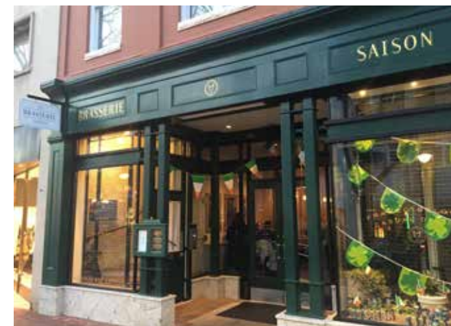
This contemporary storefront still fits within its original opening and uses traditional elements reorganized into a new design. Note the steel frames creating a transom area and the dual steel rectangular columns supporting the recessed entry.
