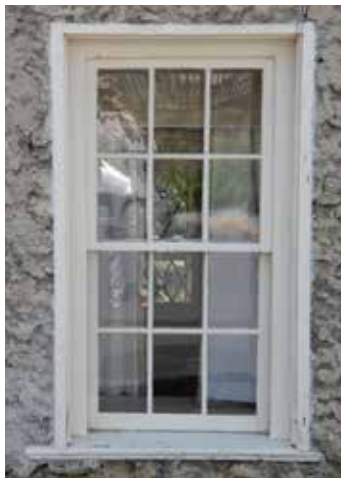
Six-over-six sash in an early 19th c. stone/stucco building.
