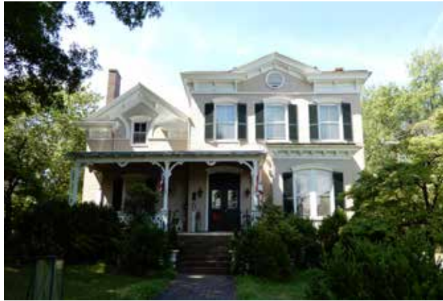
This Italianate residence with its shallow gable roof and bracketed cornice also has brackets on its porch and addition.
