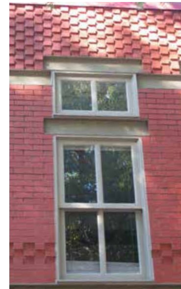
The brick checkerboard detailing and steel lintels along with the new window arrangements are contemporary re-interpretations of historic elements on this Washington, D.C. new building.
