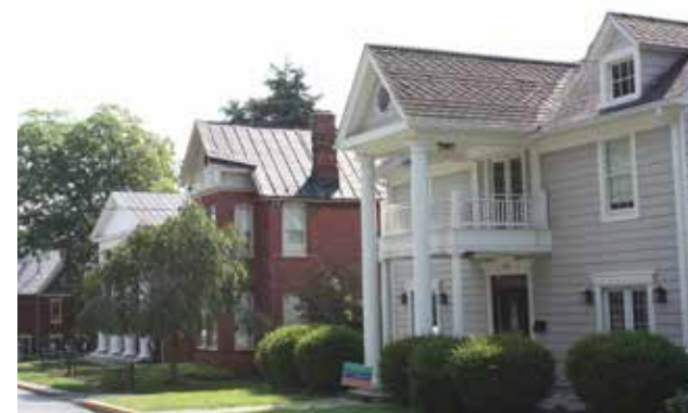
The residential districts have more variety of styles and forms, but their setbacks and heights are similar.
