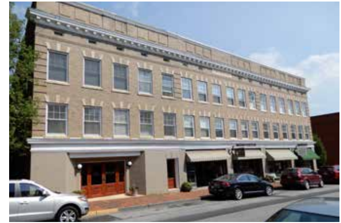
The commercial example of the Colonial Revival has several typical elements including its modillion block cornice, flat jack arches with cast stone keys, six-over-one windows and brick end quoins.
