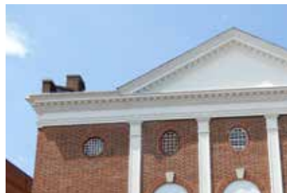
This classical cornice and pediment contain rows of dentils.
