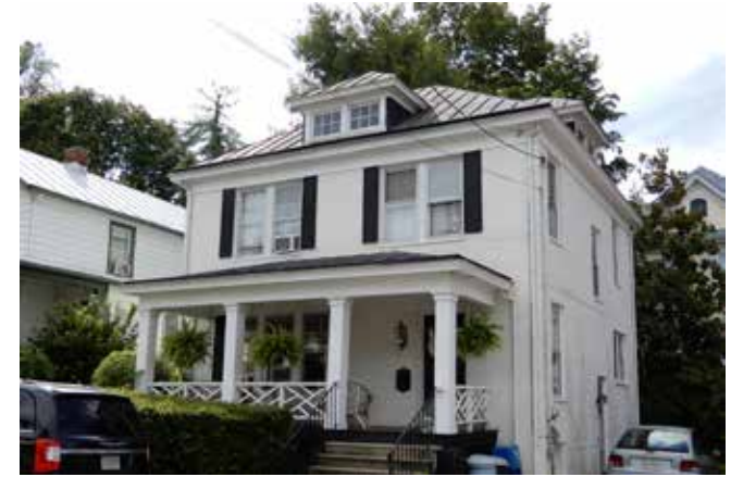
This American Foursquare is a larger example with double windows on the second level and a larger window on the main level. The shutters and railings are later changes.
