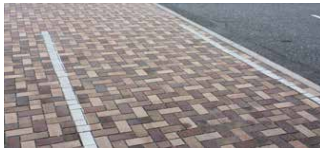
Permeable pavers are used with contrasting bricks to divide the spaces in this parking lot. This design helps reduce water runoff & the pavers are a more appropriate material than the asphalt paving.
