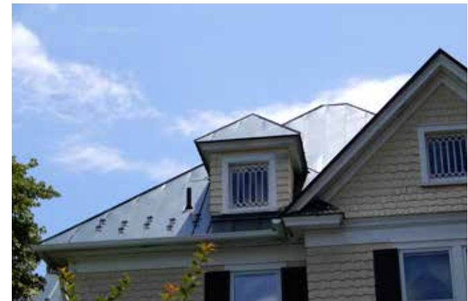
Dormer windows with a variety of decorative sash are found throughout the districts such as these diamond-pane examples.
