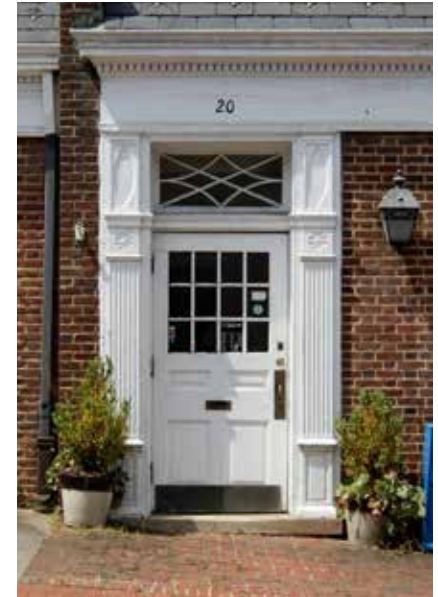
Single Colonial Revival commercial door with decorative tracery transom and multi-light and multi-panel door.
