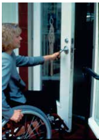
Changing hardware is a low-impact means to help create accessibility to historic buildings.
