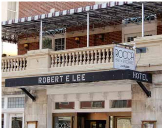
This small canopy provides entrance protection as well as a space for the building signage.
