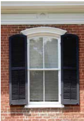
Two-over-two sash in a late 19th c. brick building. The upper sash has a segmental arch.
