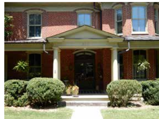
This classical portico is a well-designed, later alteration, to this Italianate styled residence.
