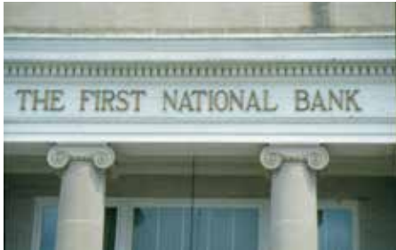
Wall signs should fit the architecture like this bank sign located in the frieze of the classical entablature.
