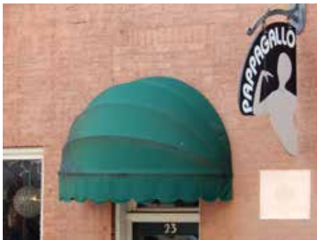
A rounded dome-shaped awning fits well over single entrances and provides an attractive highlight to a business entrance.
