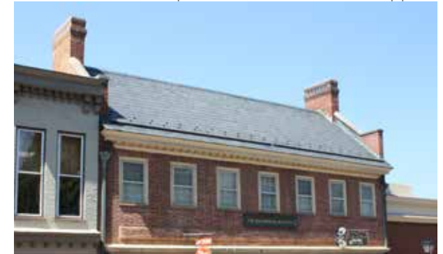
These single interior end chimneys are incorporated into the walls of the building.
