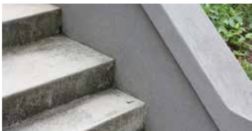
Stucco can also be applied over a masonry base to create a different appearance than brick or concrete blocks.
