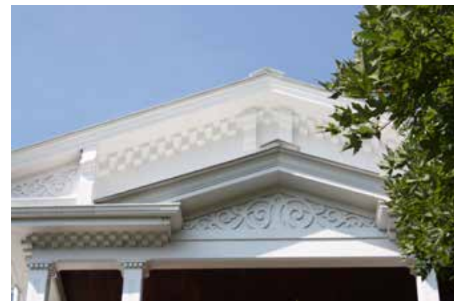
Traditional classical wood detailing is further enhanced with decorative scroll work in this example.
