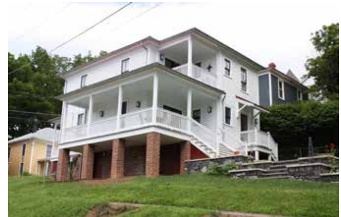
This new porch addition was placed to the side & rear of the historic house & was designed to complement the existing design & take advantage of dramatic views.
