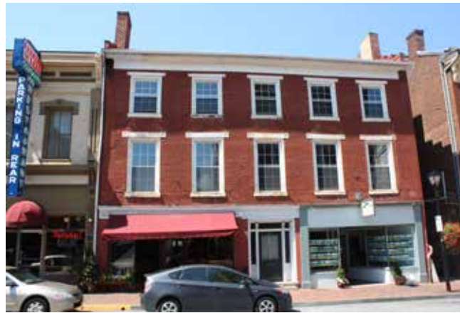
This early 19th century brick structure reflects Greek Revival details with the lintels and cornerblocks over the windows and a central entrance with transom and sidelights.
