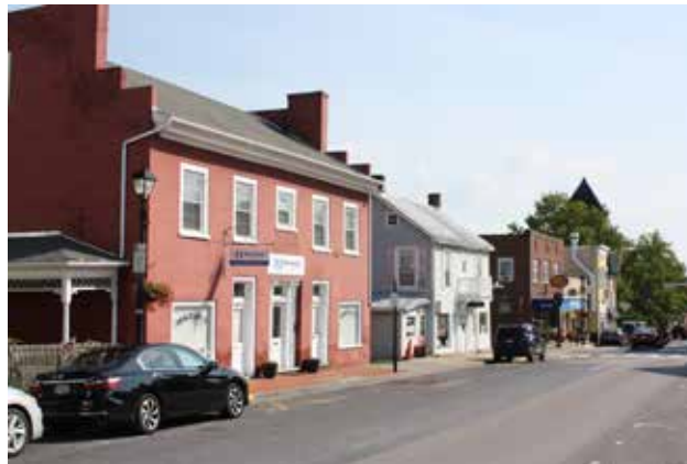
Gable-roofed early 19th brick structures add variety to typical Main Street commercial buildings.
