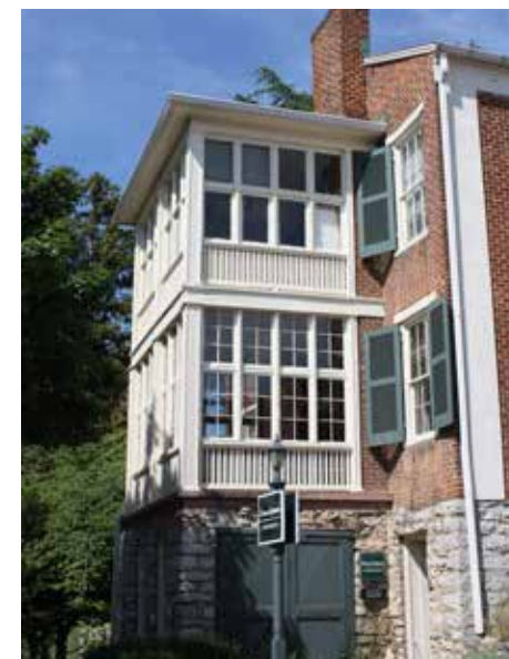
This two-story side porch appears to have originally been open and later enclosed with multi-light and single-light windows.
