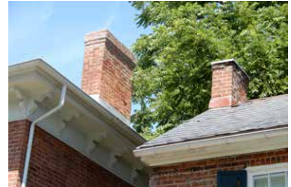
A pair of exterior end chimneys; the taller example has a corbelled cap while the smaller one is capped.
