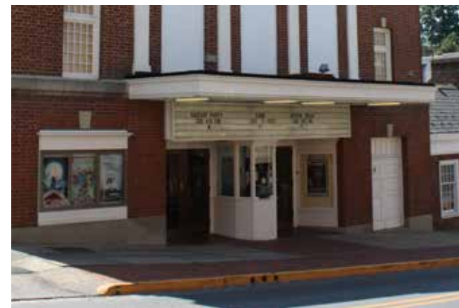
The State Theater has a projecting flat canopy and the marquee signage is a flat wall sign.
