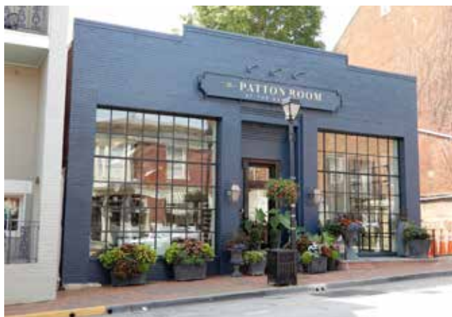
This 20th century building’s storefront was recently replaced with industrial type metal framed windows that better reflect the original garage openings of the facade.
