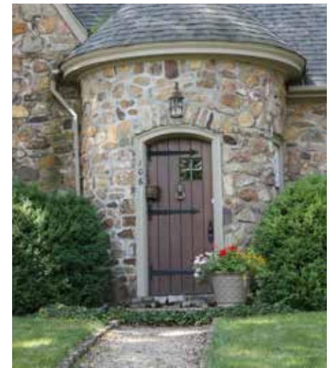
A solid-door in a Tudor Revival style house with large hinges and vertical wood planks.
