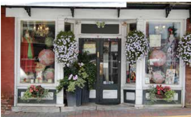
Early wood storefront with double wood doors.
