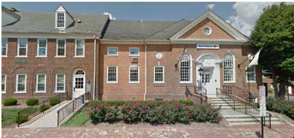
Because these buildings are set back deeply from the sidewalk, an accessible entry ramp was easily accommodated to the main level of the building.
