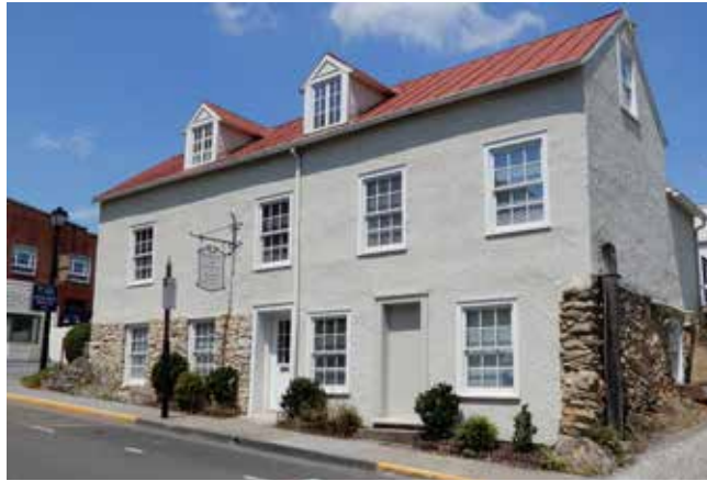
This early example of a vernacular Federal era structure is constructed of stone and stone covered with stucco.
