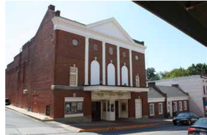
This theatre has a false front central pediment supported by four pilasters. Its three large arched openings reflect an Italian influence of a piano nobile level above the lower entrance.
