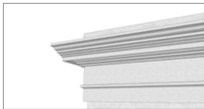
A typical three-part entablature consisting of the cornice, frieze, & architrave (from top to bottom).
