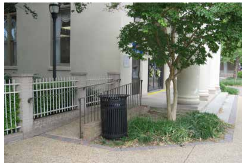
The setback and side yard space of this example allowed for a side ramp to be installed to the front portico entrance.
