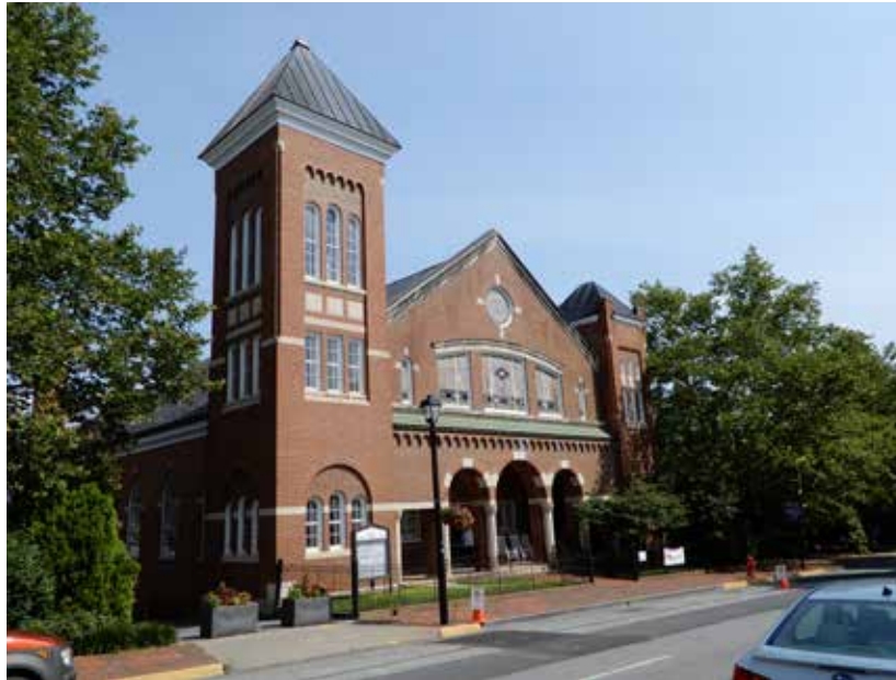
Sets of triple arches at its recessed entry and in its adjoining tower help identify this Romanesque Revival church.
