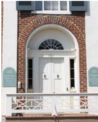
Arched entrance with double-paneled doors, an arched fanlight and sidelights.
