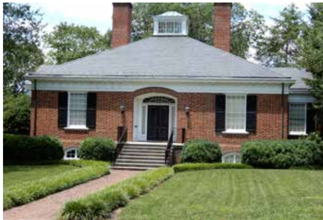
A more recent example of the style executed in a one-story plan with a very prominent hipped slate roof containing a central lantern and very tall brick chimneys. The central entrance segmental arch is repeated in the cornice. Note the elliptical fanlight transom and sidelights.
