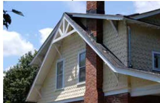
The decoration on the gable end of this bungalow includes brackets and a framed gable detail.
