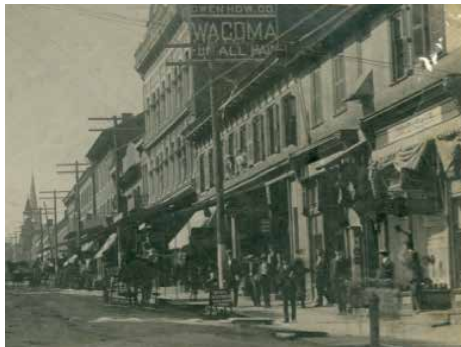
This historic image shows the popularity of awnings on the south-facing buildings on Main Street. The awnings were a key feature in reducing heat gain & glare on the storefronts & window displays while also providing shade for customers.
