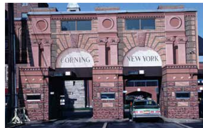
Here a drive-thru addition on the rear of a historic bank building is treated to a trompe l’oeil (trick of the eye) technique. The mural reflects a Romanesque Revival style with large arches and stone bases, all executed in paint on a flat surface. Different colors and shadow lines add to the realistic 3-dimensional effect on an unadorned addition.
