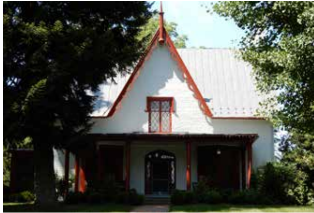
This typical example of a Gothic Revival cottage has the steep pitched roof with a central gable and decorative bargeboard and finial. A pair of diamond paned windows with a hoodmold is a typical detail.
