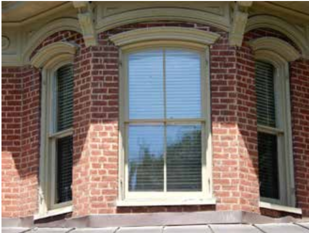
Bay window with two-over-two sash with arched upper sash and window hood.
