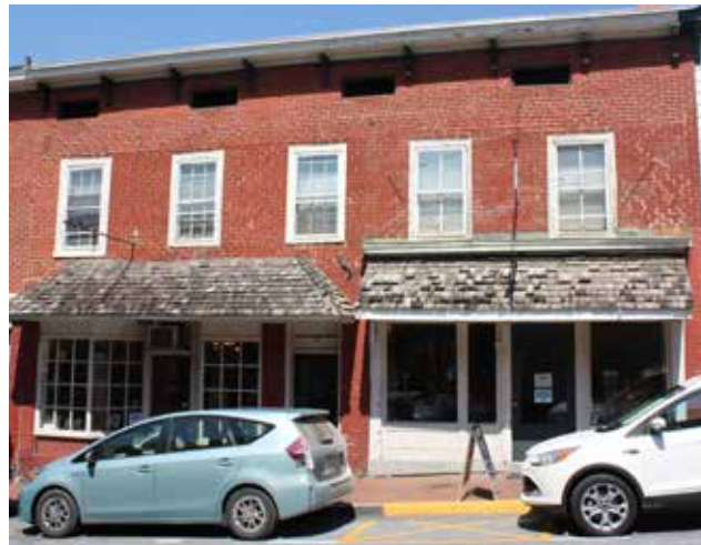
Mansard roofs with shingles or metal have been added over time to several commercial buildings in Lexington's historic districts. Original transom windows may still exist in some cases.
