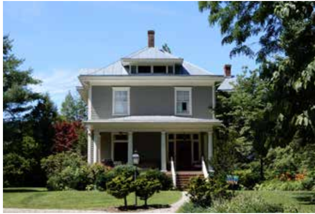
This trademark example has the square proportions, hipped roof, a large central hipped dormer and a full-width front porch.
