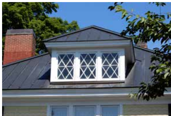
Dormer windows with a variety of decorative sash are found throughout the districts such as these diamond-pane examples.
