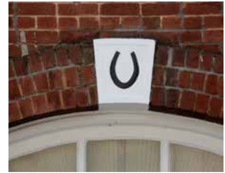
Masonry keystone with horseshoe cutout on segmental arch.
