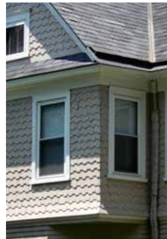
One-over-one sash in a Queen Anne house.
