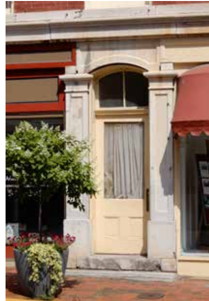
Historic door with upper single light and two lower wood panels. This door provides access to upper stories.
