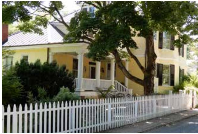
This low picket fence defines the side lawn of this historic property; its interior horizontal rails are correctly placed.
