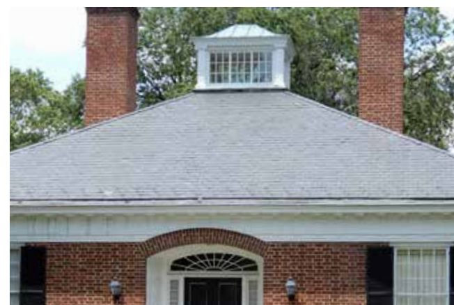
Another example of a visually prominent slate roof is seen on this hipped example of the Colonial Revival styled residence.
