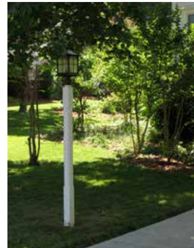
Wood is also used as the pole for some residential site lighting as seen in this example.
