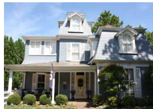
A second example of the Mansard with its dormers, projecting bay and partial wrap-around porch.
