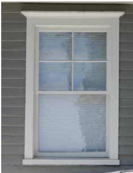
On frame buildings, windows & doors are typically surrounded by trim raised from the surface of the siding.
