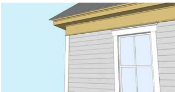
Residential cornices may be simple, like this example or more elaborate; it generally depends on the style of the house.
