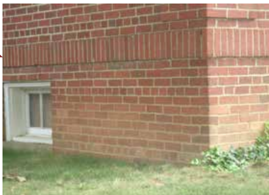
On this brick building the foundation is also brick but is articulated with a soldier course.
