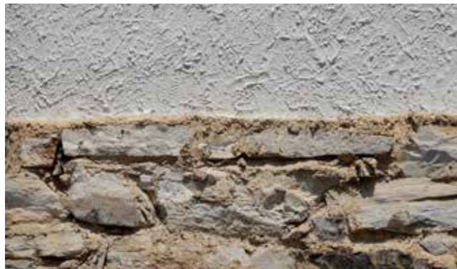
Native limestone is a prominent building material used for retaining walls & building foundations. This example has limestone rubble as the foundation with a stucco wall above.
