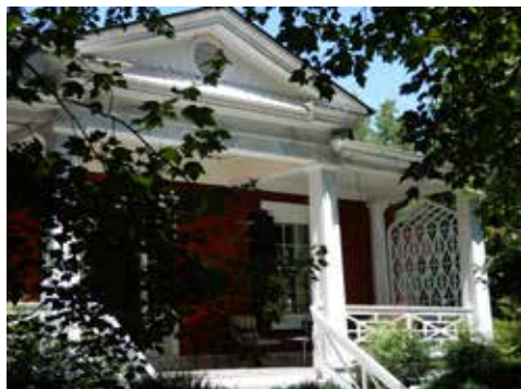
This classical porch is one-story with a projecting portico incorporated into the porch roof. Note the Chippendale railings and Tudor arched decoration.
