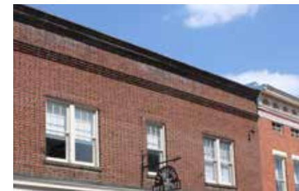
This example of a brick cornice has a flat band of brick supported by corbelling.
