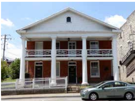
This full-length classical portico, with four Roman Doric columns, has a second floor balcony with Chippendale railings.
