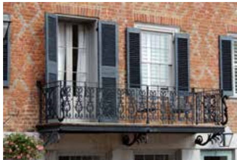
A decorative cast iron railing adds a historic detail to this small balcony.
