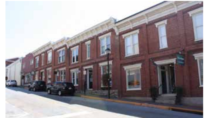
This block of Washington Street steps down the street with unified brick facades and bracketed cornices creating a street wall.
