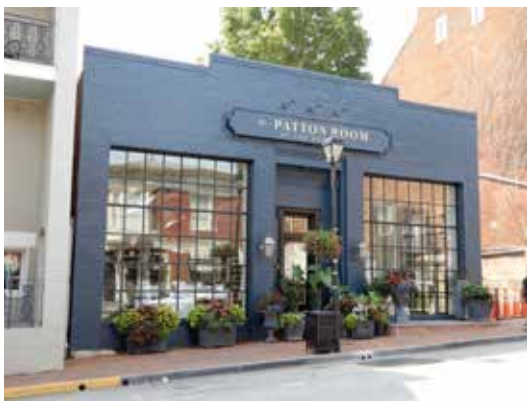
Early 20th c. storefront with essential elements. As often happens over time, the transom glass has been painted over.
