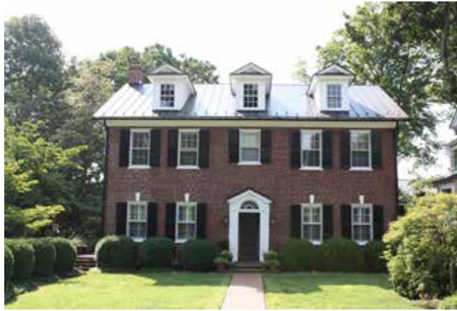
This five-bay, Colonial Revival, brick dwelling has a symmetrical facade with six-over-six windows capped with jack arches and keystones. Three gable-roofed dormers and a central entrance with an arched fanlight within its pedimented surround complete this orderly composition.
