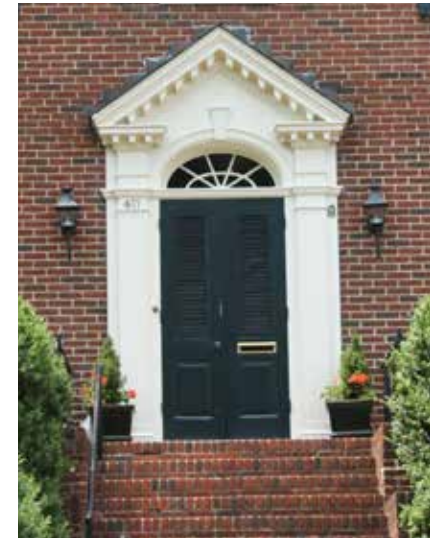
A carefully designed & fitted pair of paneled & louvered storm doors on a Colonial Revival styled entry.
