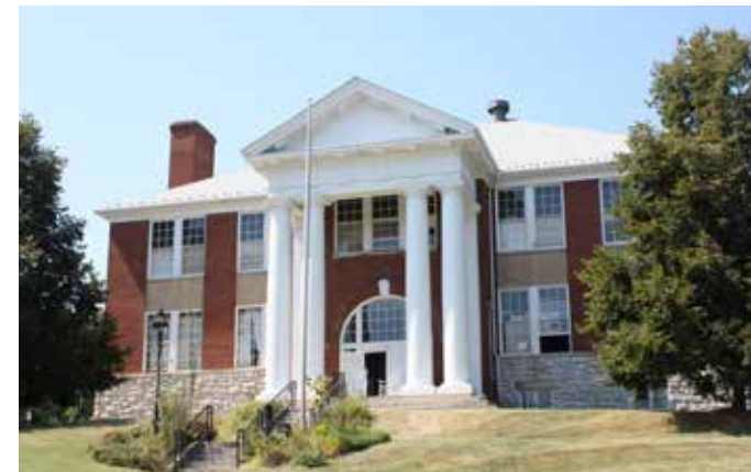
This Classical Revival former schoolhouse has a very prominent central portico supported by Roman Doric columns. Paired windows in six-over-six patterns are typical of the period.
