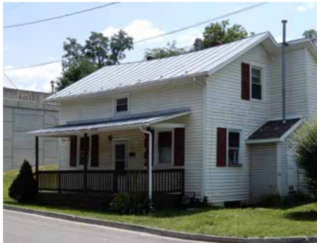
A typical vernacular frame cottage with a shed-roofed porch and minimal decoration.
