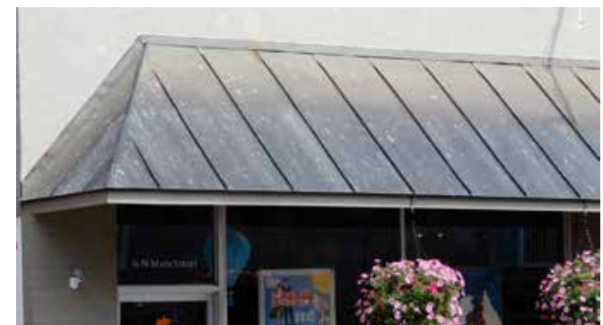
Mansard roofs with shingles or metal have been added over time to several commercial buildings in Lexington's historic districts. Original transom windows may still exist in some cases.
