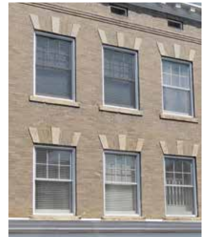
Colonial Revival style windows can have a variety of multi-paned and single-paned sash.
