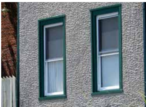
Stucco was used as a wall cladding in the late 19th c. & early 20th c. on various styles of architecture.
