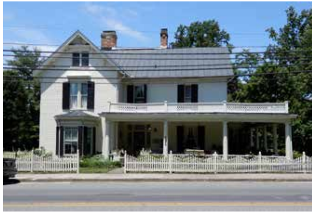
This typical example is an “L” shaped frame dwelling with its wrap-around porch and front bay window.
