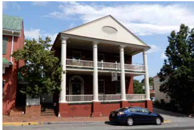
The Wilson-Walker House has a temple front with the trademark two-story portico and Roman Revival columns. When Main Street was lowered its brick foundation was exposed and rebuilt.
