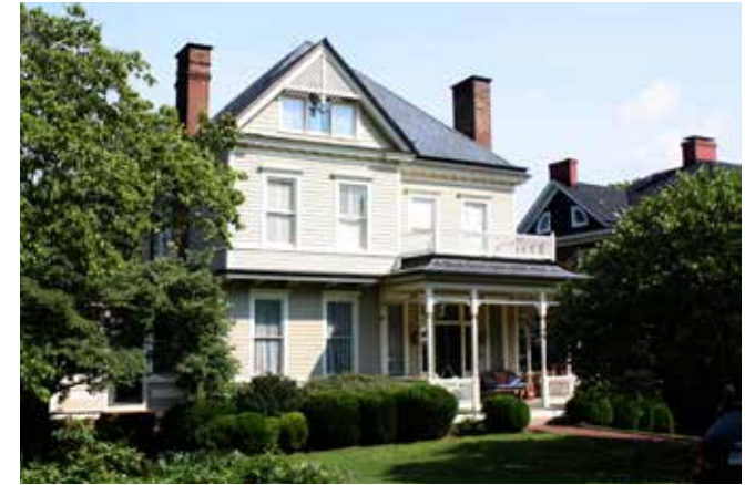
This Queen Anne house has a projecting decorative gable with a partial wrap-around porch. Its tall chimneys have decorative corbels.
