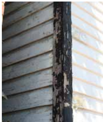
Exposed wood will rot quickly without proper preparation & painting with a primer & two top coats of paint.
