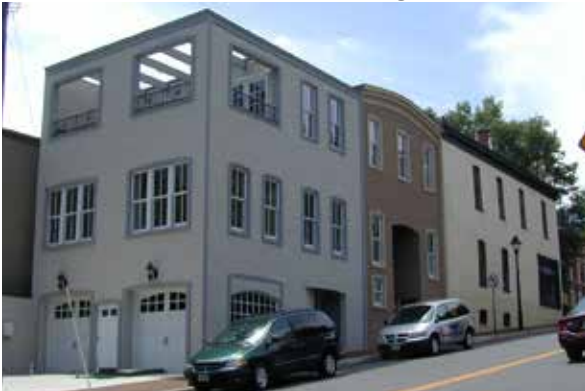
The new, two-part, rear addition on this Warrenton, VA building respects the height, materials, & width of the historic building while having a contemporary 3rd floor balcony & 1st floor garages.
