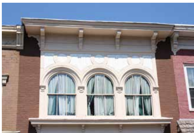
This commercial facade is embellished with finely crafted wooden wall surface decorations, cornice brackets, and window trim.
