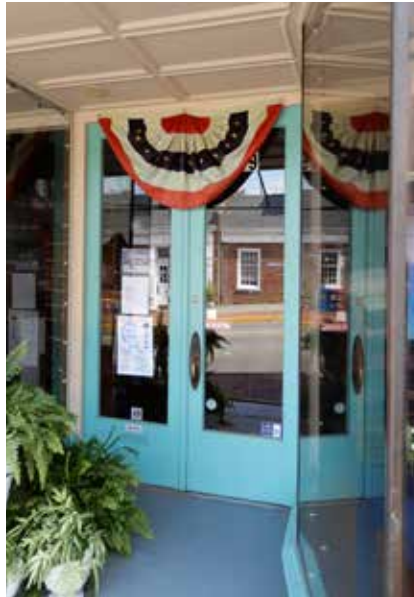
Typical commercial single-light wooden door, in this case a double door within a recessed entryway.
