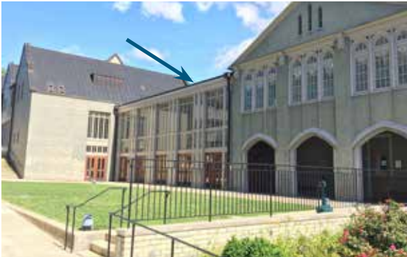
The glass connector successfully attaches the new addition (rear) to the historic building (front).
