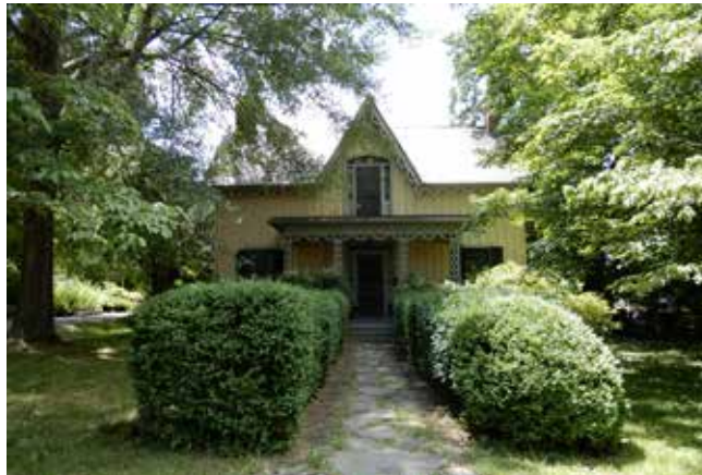
Another example of the Gothic Revival cottage with its central decorative gable is executed in board-and-batten. The front veranda is similar to the example above.
