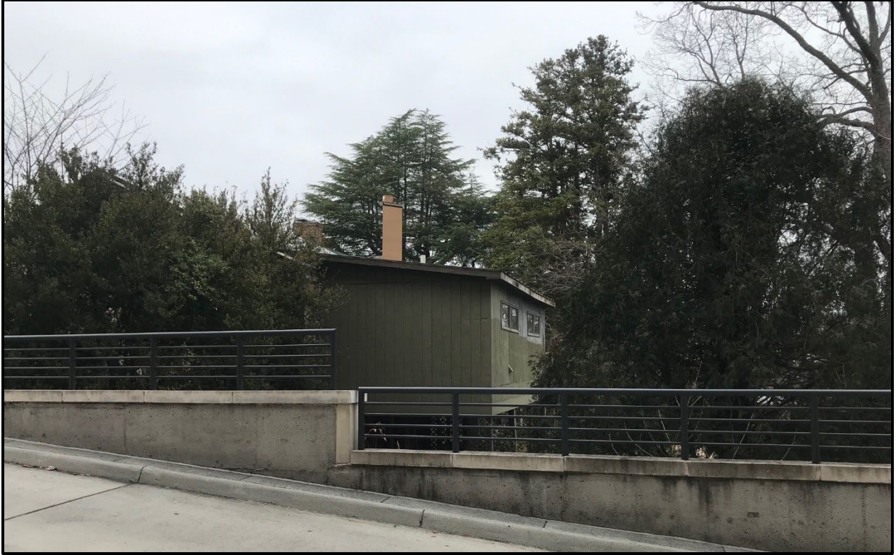
10 South Randolph Street with full-scale mock-up chimney
