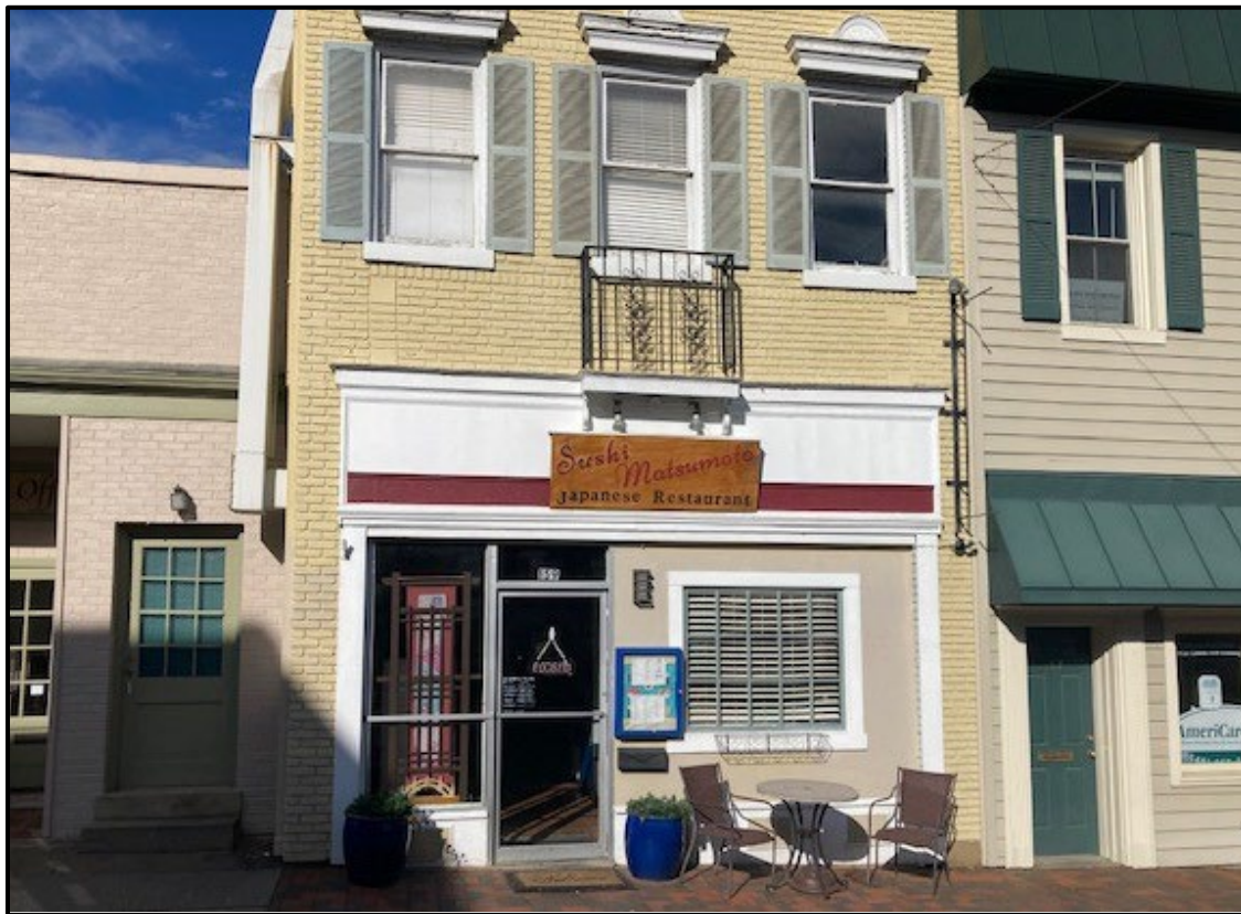
159 S. Main Street existing conditions
