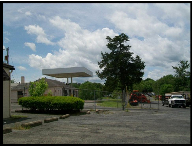
At site facing west from Transportation building parking lot
