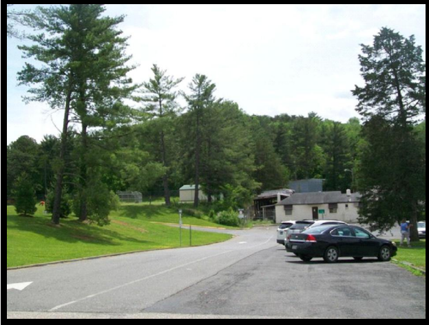
North of site facing southeast from Waddell Street
