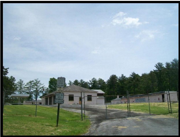
At site facing southeast from gravel road
