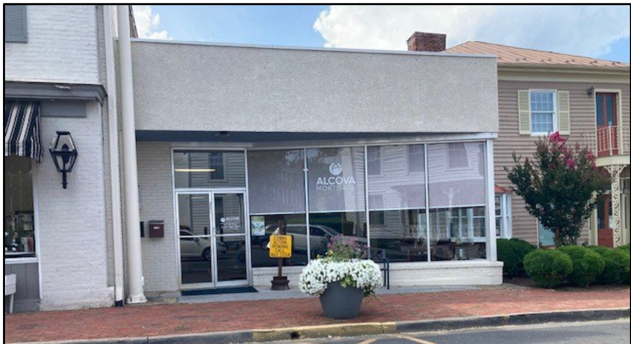
photograph of front of 221 South Main Street
