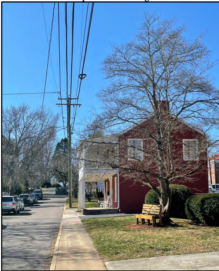
205 S. Randolph Street existing conditions
