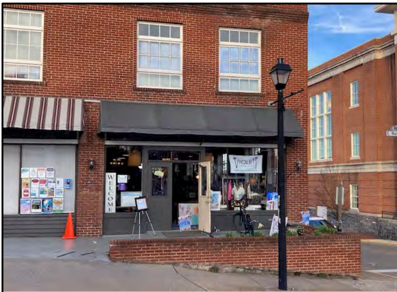
18 E. Nelson Street existing conditions
